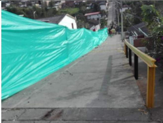
Cerramiento tramo 5R, 7R, 5ALL, 1ALL
